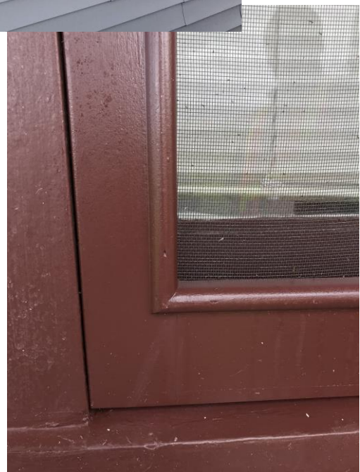
Photo right: Close-up view showing the detail of the fiberglass screen frame.
