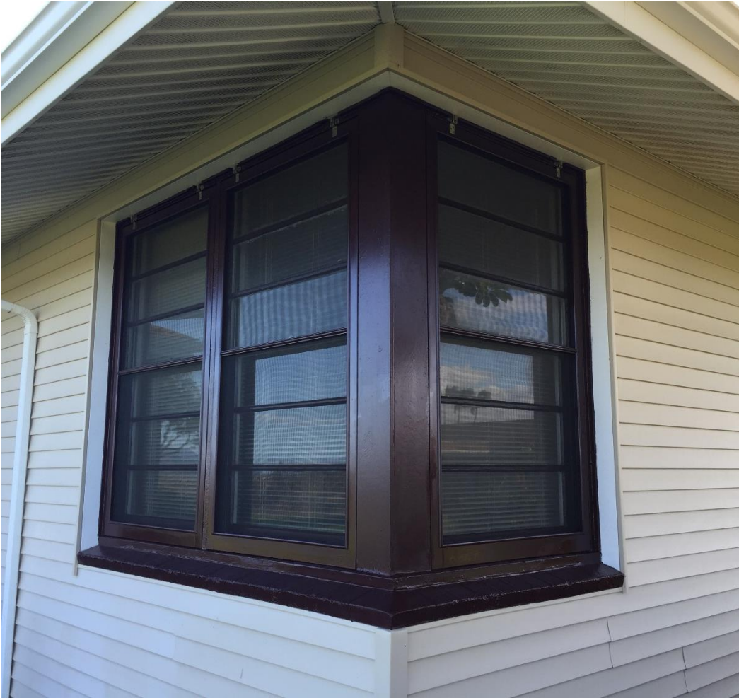
Photo above: Heleloa window repaired with new fiberglass framed screens.
